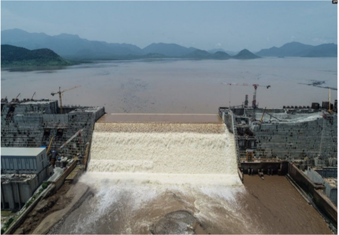
Figure 8.1 The Under Construction of the Grand Ethiopian Renaissance Dam, (source: countryhighlights.com)
